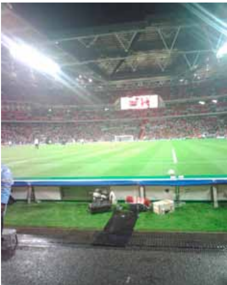
HAURATON SERVICE CHANNELS at Wembley Stadium in the UK
