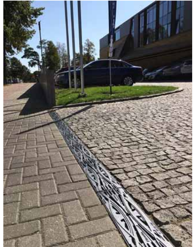
KTL corrosion resistant finish on METROPOLIS ductile iron grating
