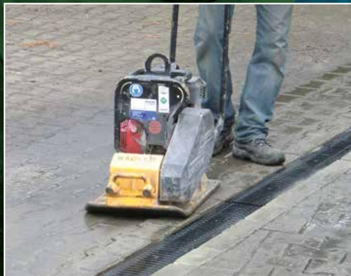
Elasticity is important when permeable paving surfaces are being compacted in along the **RECYFIX** channel.
