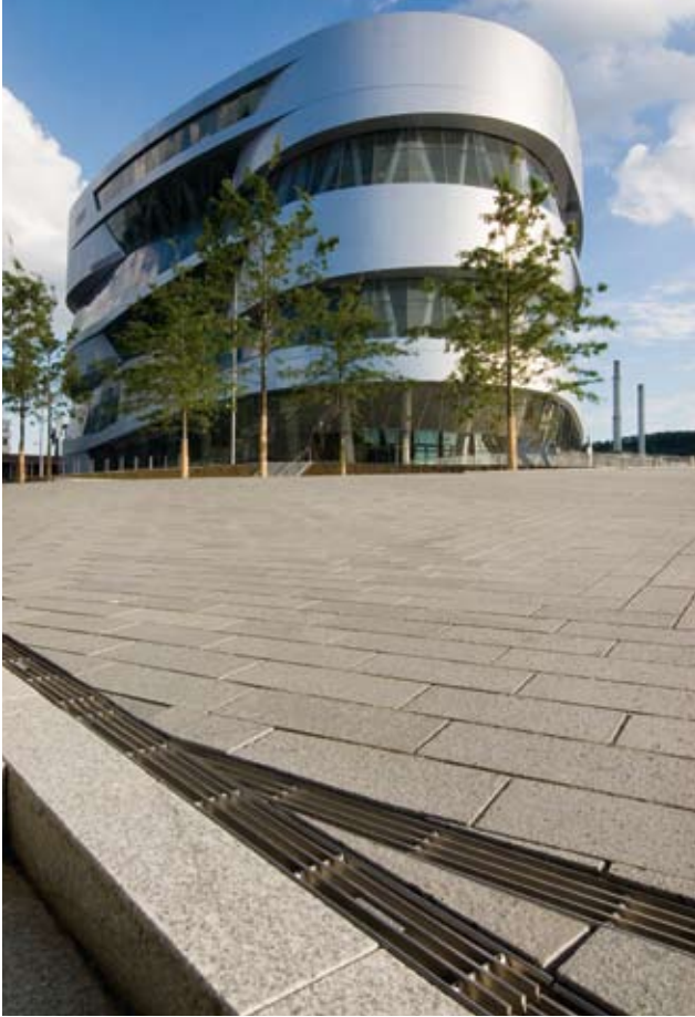
The stainless steel drainage channels were developed according to site-specific requirements.
