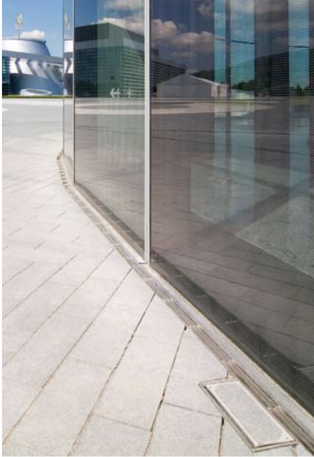
Water from the façade is drained via channels with longitudinal grating and removable sidewall. Special inspection boxes allow access to the channels for servicing.
