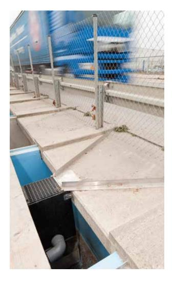
**Rainwater treatment with filter substrate channel.** Systems for the effective and ecological treatment of rainwater.
