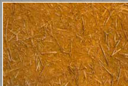
Clay wall reinforced with plant fibres.
