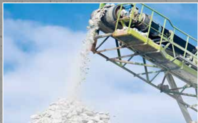
Concrete recycling, re-use e.g. in road construction.
