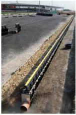
After over 10 years of use, the RECYFIX HICAP channel runs at Doncaster have provided trouble-free drainage with no failures reported in any of the components installed.
